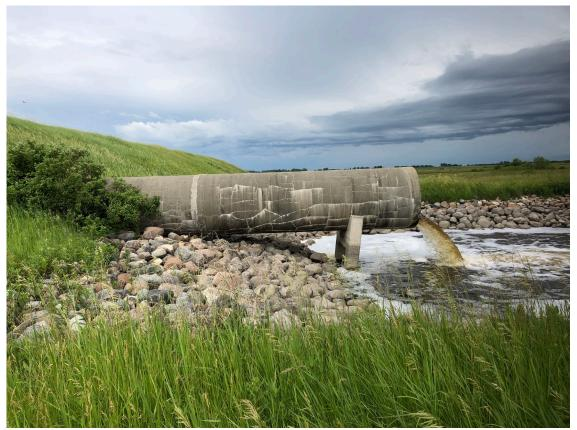
Pipe prop tilted. Appears no worse than when first identified. Wood vegetation to be removed 2022
