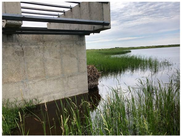
Inlet west side, debris on southside of structure, removal needed
