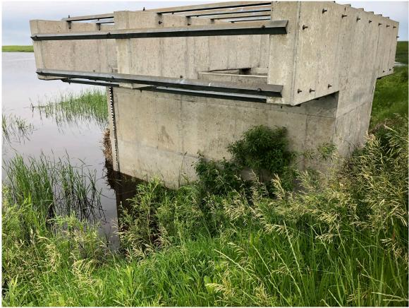
Inlet structure - woody vegetation around inlet, removal in 2022. Debris on south side to be removed
