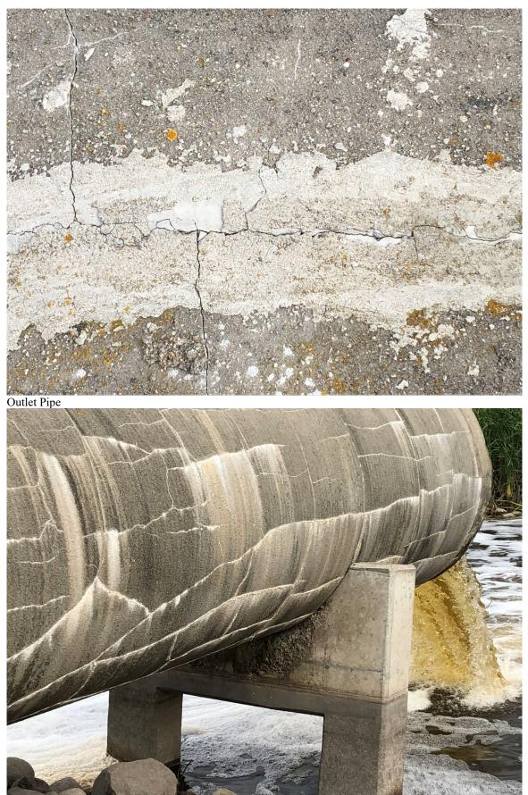
Outlet pipe cracking. Pipe is fully cradled
