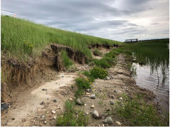
Erosion on pool side of north embankment, significantly more damage since prior years
