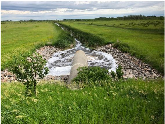
Pipe outlet - riprap plunge pool. WD will remove woody vegetation on embankment and in rock in 2022
