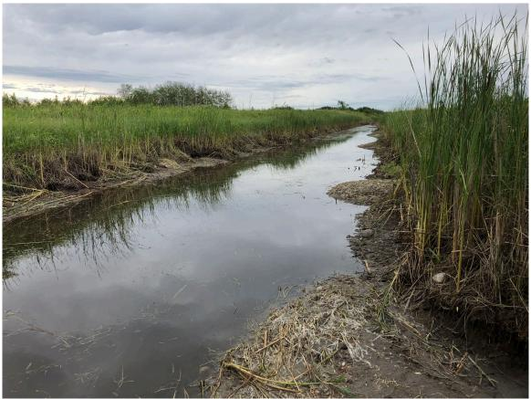
End of outlet channel looking east, erosion along banks
