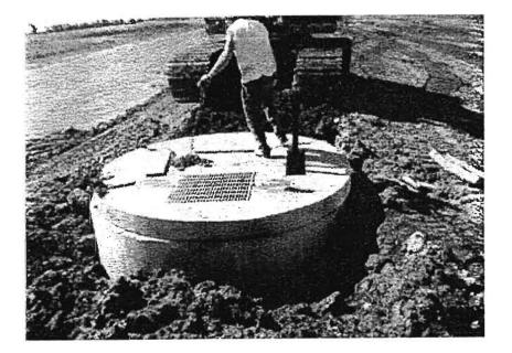
Photo 7: Station 19+50. Installation of cover on principle outlet.
