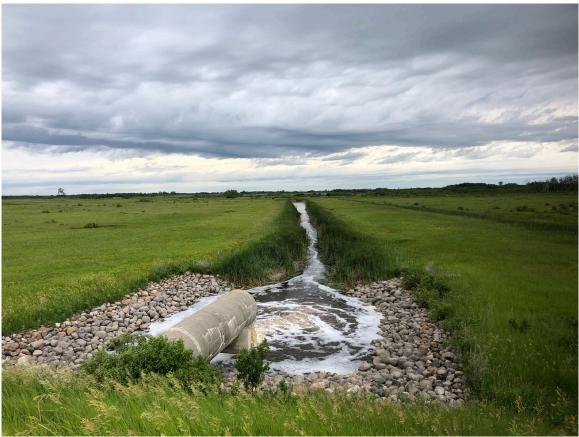
Outlet pipe and channel, obstruction visible at outlet channel
